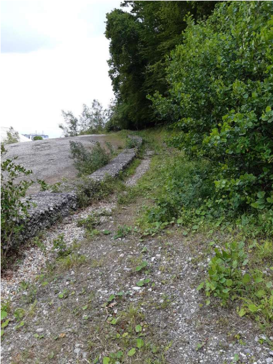
Photograph 3 – Gabion wall and French drain, south side of Old Works area
