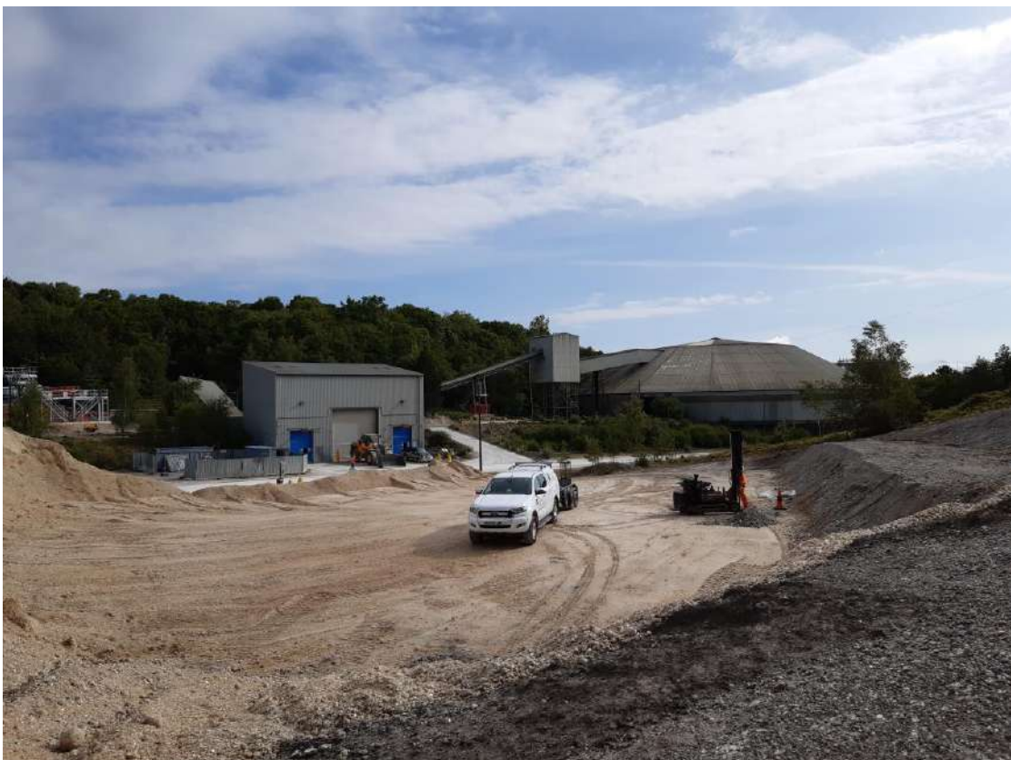
Photograph 2 – view north east across the site
