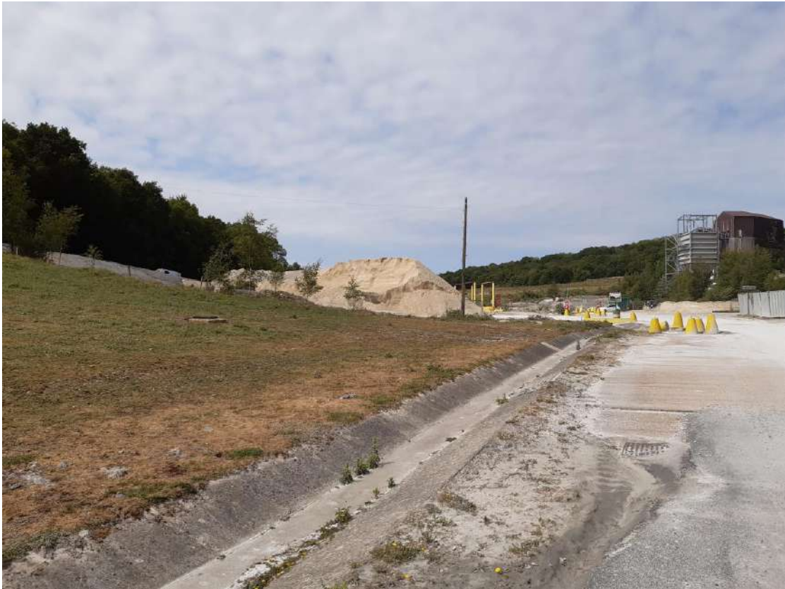
Photograph 1 – Existing channel drain beside access road
