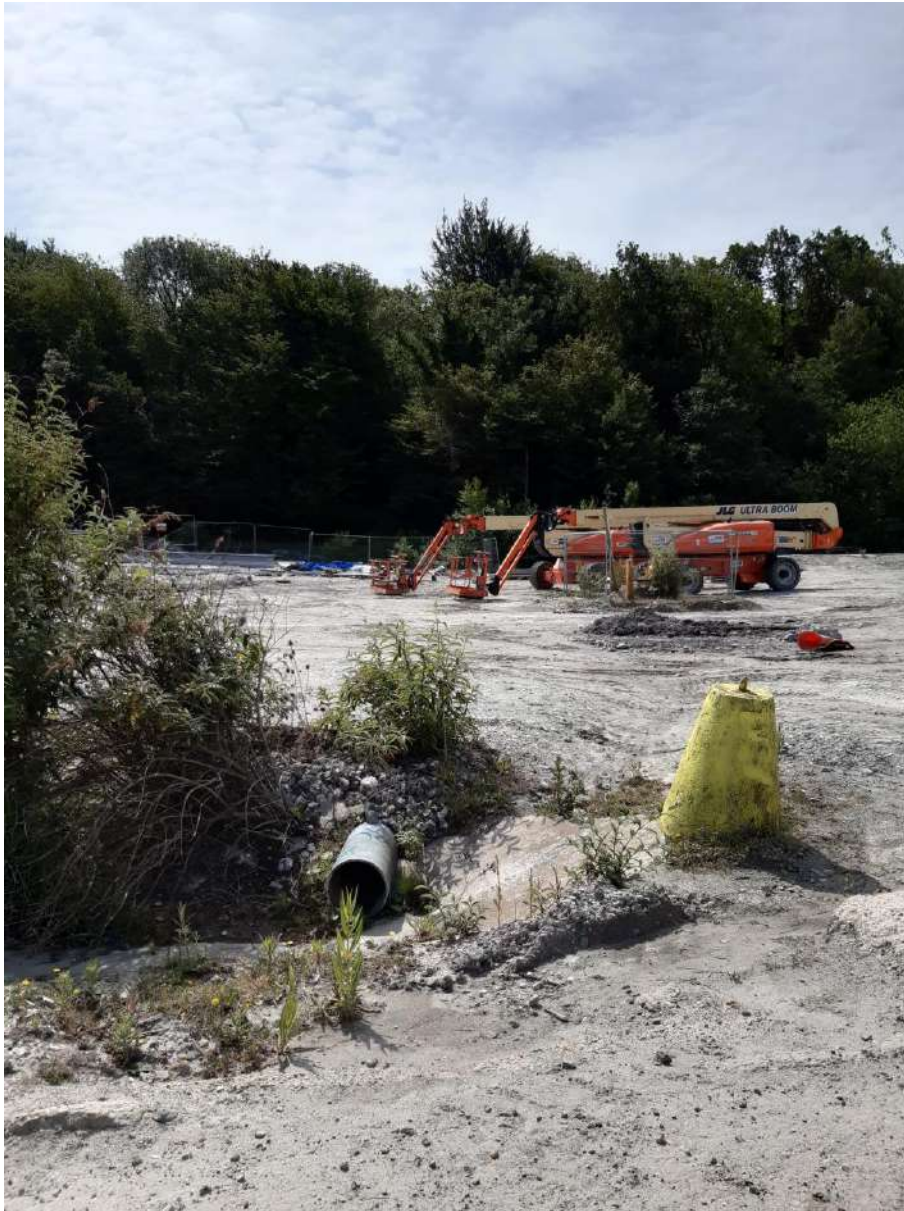
Photograph 4 – Drainage outfall from filter drain behind south side gabion wall
